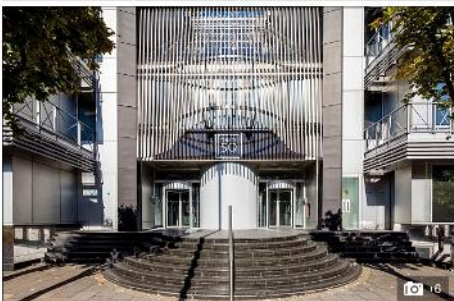
The new development is expected to attract first-time buyers as well as investors
