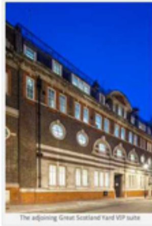
The adjoining Great Scotland Yard VIP suite.
