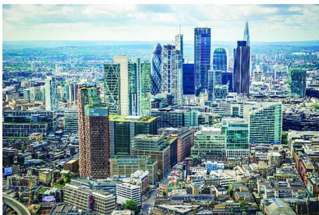
Looking east, with the development in the foreground
