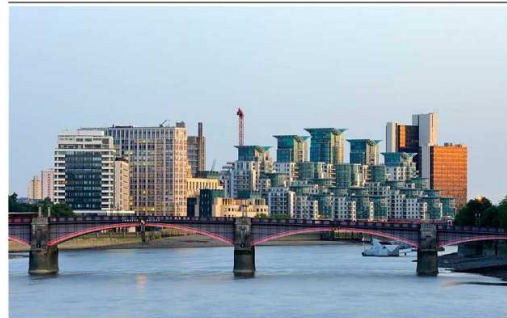
More flats on the London skyline. Housebuilder Galliard, which has 4,000 homes in the pipeline, has announced it will deliver 2,000 additional suites and apartments in London. Photo: imagebank / Alamy
